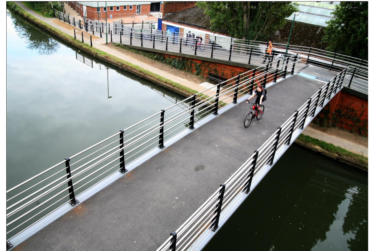
Not only did the new "Grand Union Bridge" facilitate significant improvements for pedestrian and cyclist access to the Grand Union Canal, near Alperton, it was successful in its overarching objectives and aspirations to design out crime.
